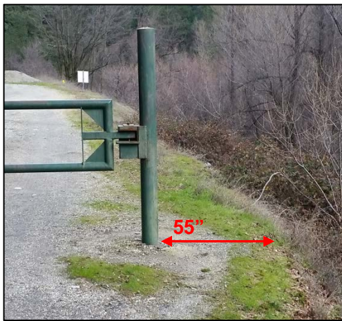
Outside Gate Opening (river side)
